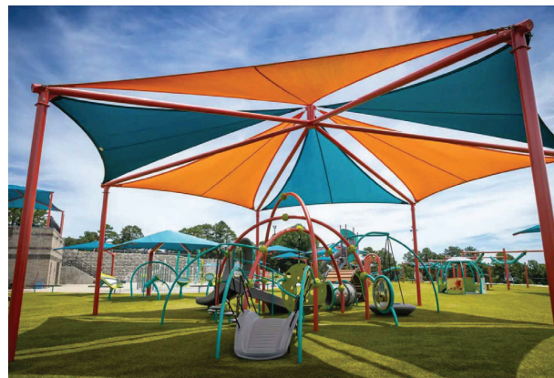
PLAYGROUND OVERHEAD SHADE STRUCTURE
