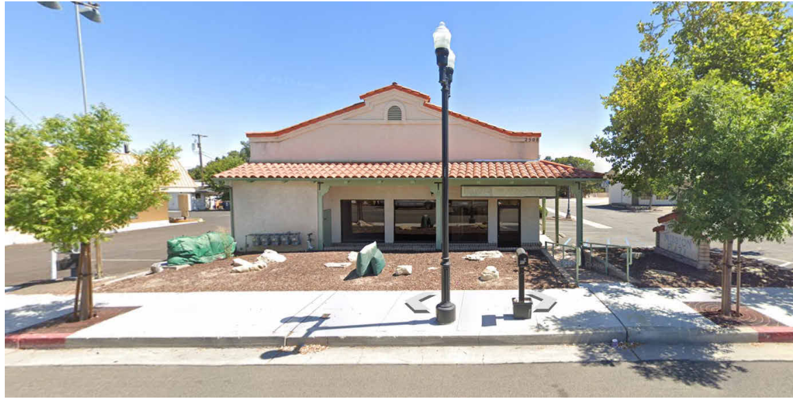
WEST ELEVATION FROM SPRING ST.
