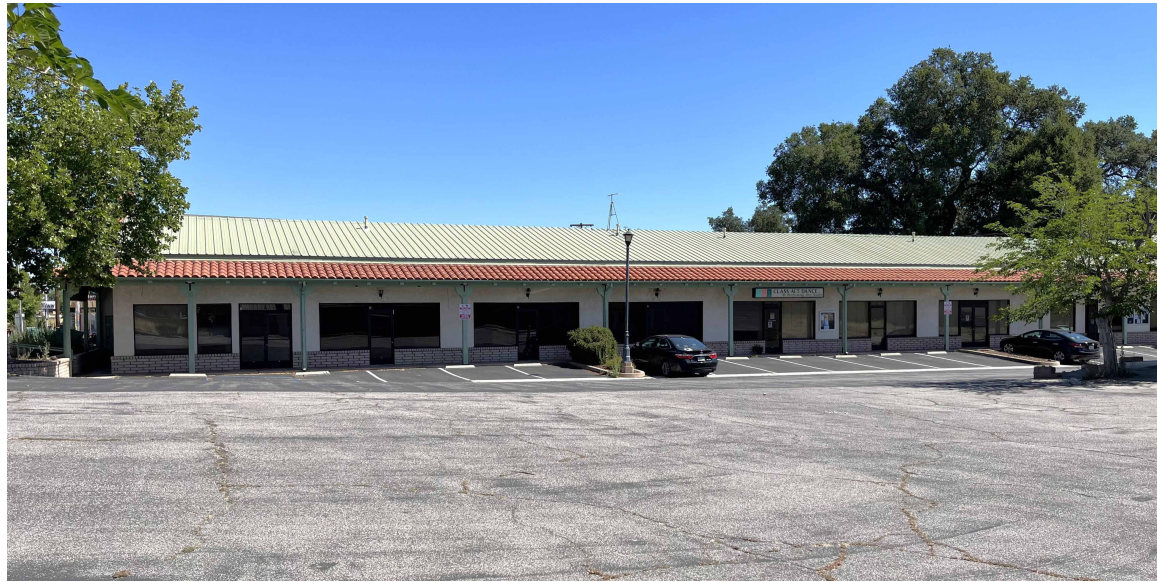
SOUTH ELEVATION FROM PARKING LOT
