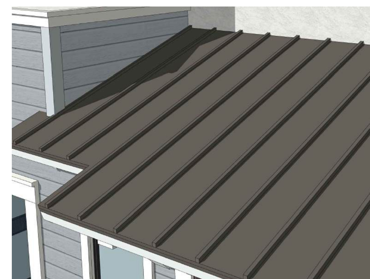
11 STANDING SEAM ROOF
