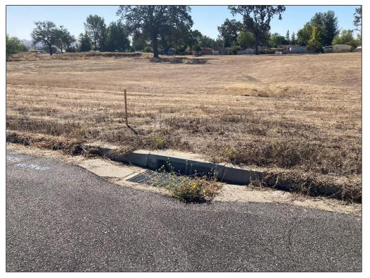
Photo 4. View from Nutwood Circle; drain leading to culvert pipe to direct flow into shallow man-made basin within the BSA (aspect southeast; 9/30/22).
