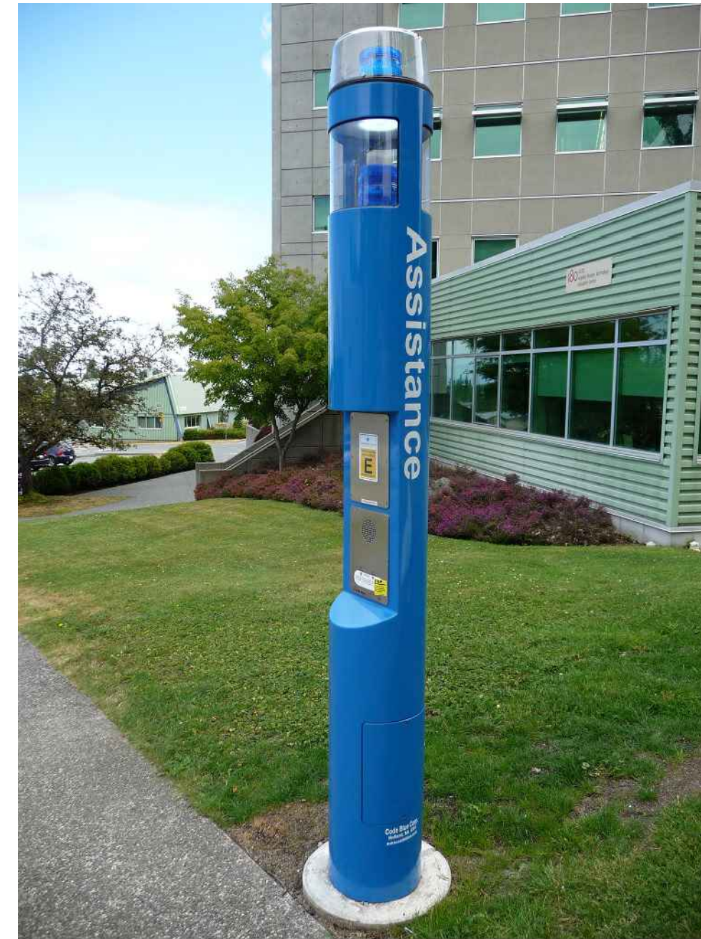
EMERGENCY CALL STATION
