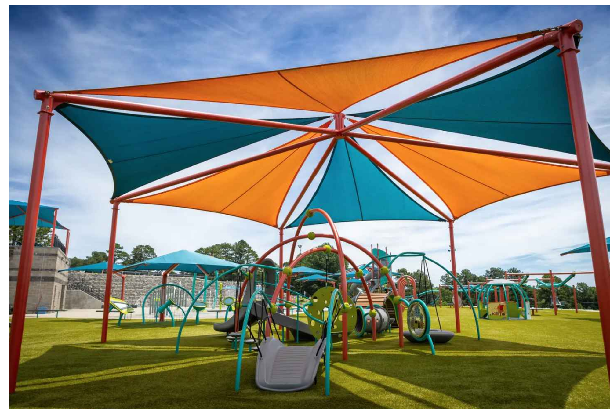
PLAYGROUND OVERHEAD SHADE STRUCTURE
