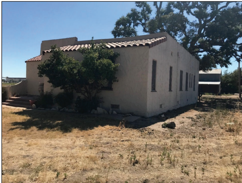
Photo No. 3: Northeast corner of B1 (residence), facing southwest. Photo taken 7/22/2019.
