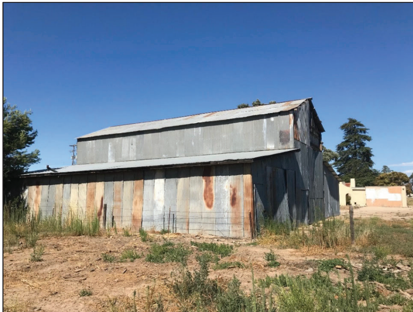
Photo No. 11: B3 southwest corner, facing northeast. Photo taken 7/22/2019.
