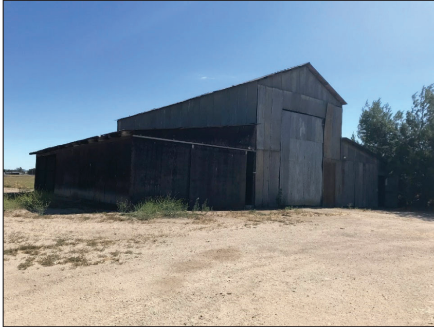
Photo No. 10: B3 northeast corner, facing southwest. Photo taken 7/22/2019.
