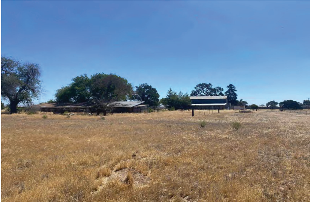
Figure 16. Overview of existing structures on project area facing Northeast
