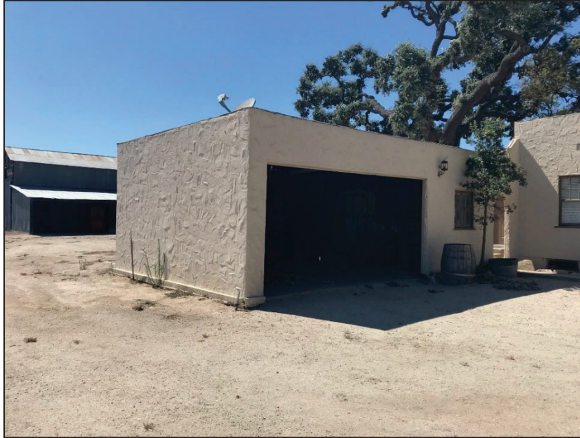
Photo No. 6: B2 southeast corner, facing northwest. Photo taken 7/22/2019.
