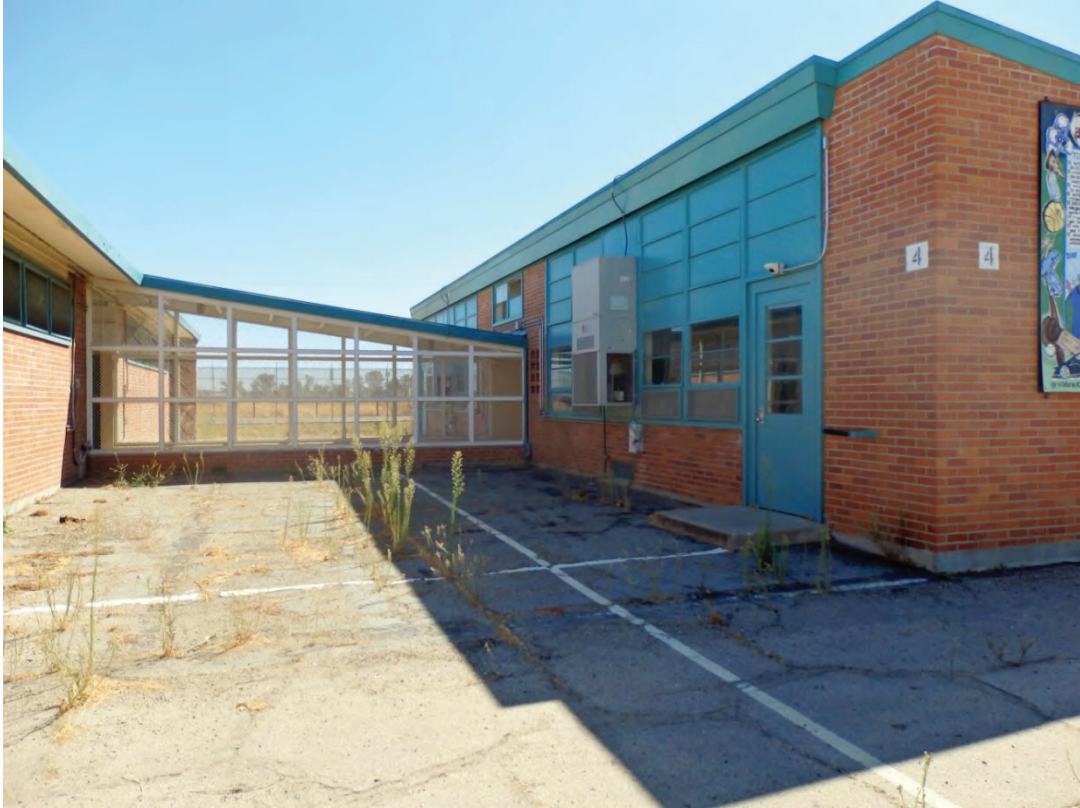
Looking east to central hallway.
