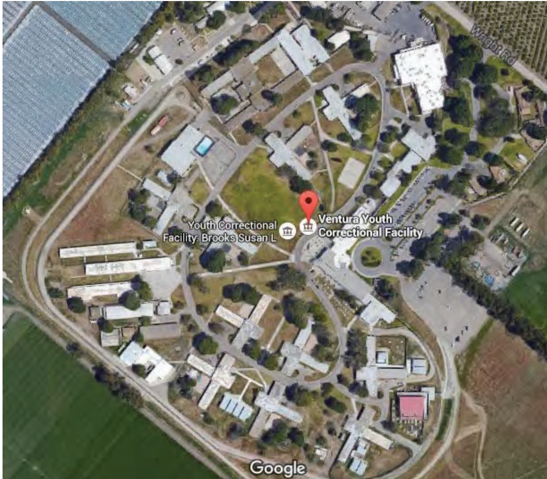
Exhibit 7. Open campus design, Ventura Youth Correctional Facility.
