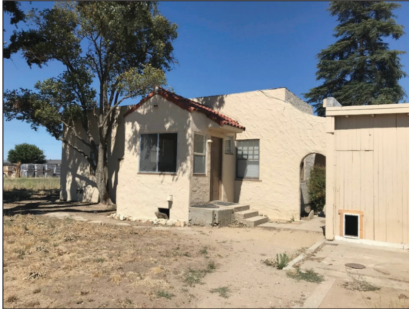
Photo No. 4: B1 west elevation, facing northeast. Photo taken 7/22/2019.
