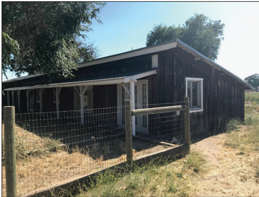
Photo No. 13: B4 northeast corner, facing southwest. Photo taken 7/22/2019.
