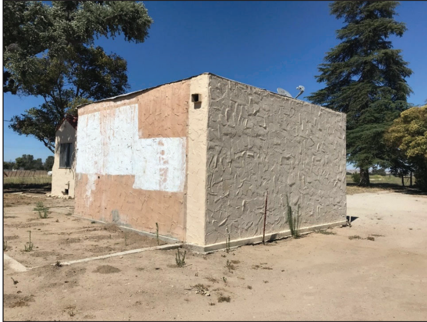
Photo No. 8: B2 southeast corner; facing northwest. Photo taken 7/22/2019.
