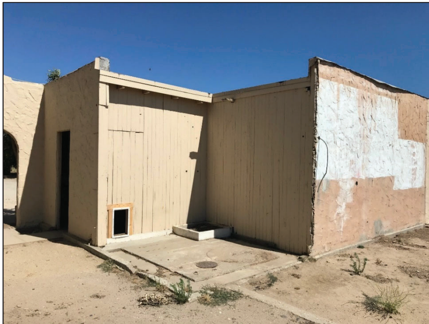
Photo No. 7: B2 northwest corner, facing southeast. Photo taken 7/22/2019.
