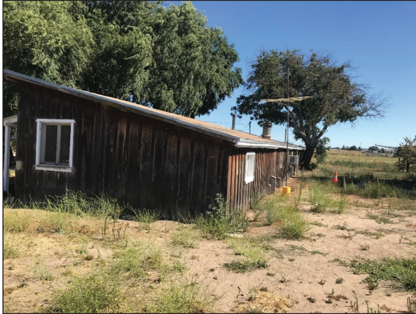
Photo No. 14: B4 northwest corner, facing southeast. Photo taken 7/22/2019.
