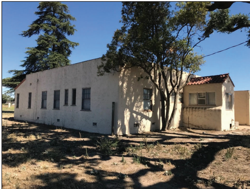
Photo No. 5: Northwest corner of B1 (residence), facing southeast. Photo taken 7/22/2019.
