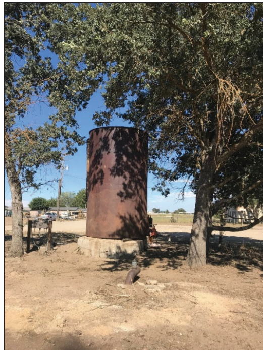
Photo No. 15: S1, facing east. Photo taken 7/22/2019.
