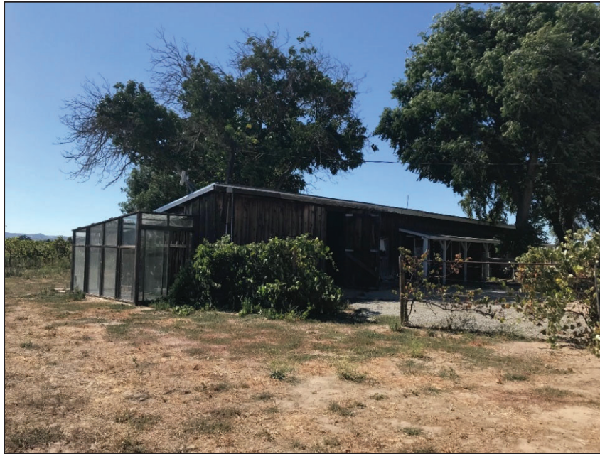
Photo No. 12: B4 southeast corner, facing northwest. Photo taken 7/22/2019.
