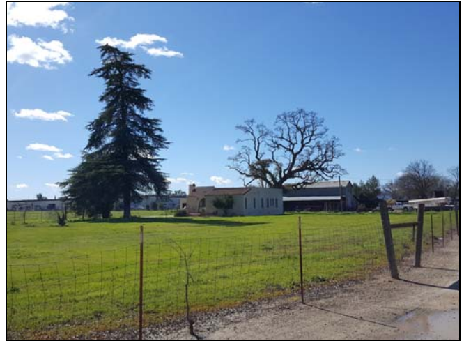
Photo 2: View of the residential structure built in 1928 near the northeast corner of the property.
