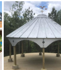
SILO SHADE STRUCTURE
