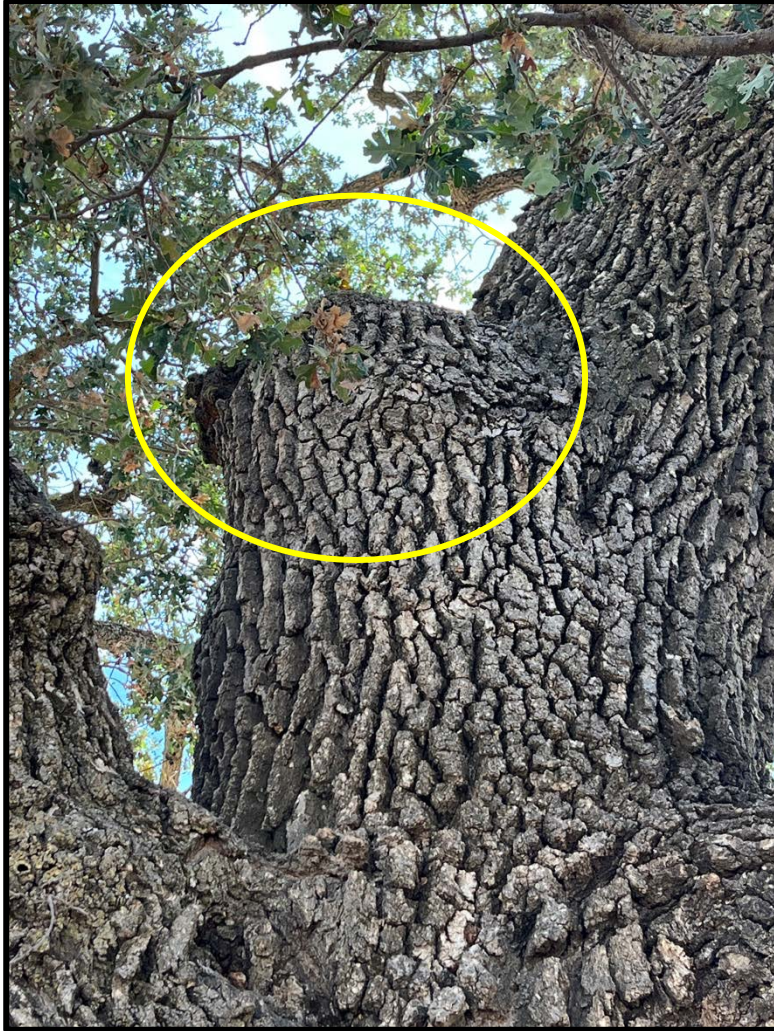
Photo 9 - Tree 2 with decay cavity formed by failed scaffold circled at center of tree, approximately 14 feet above ground.
