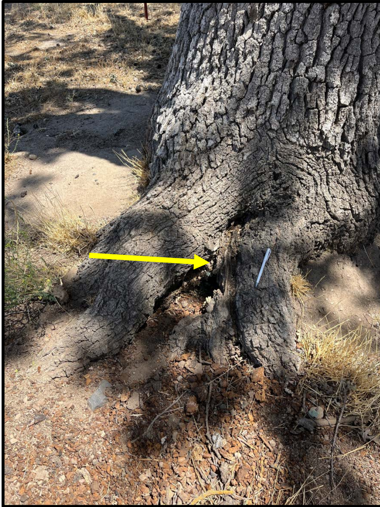
Photo 2 - Tree 1 with decayed anchor root on southwest side, indicated by arrow. Ink pen provided for scale
