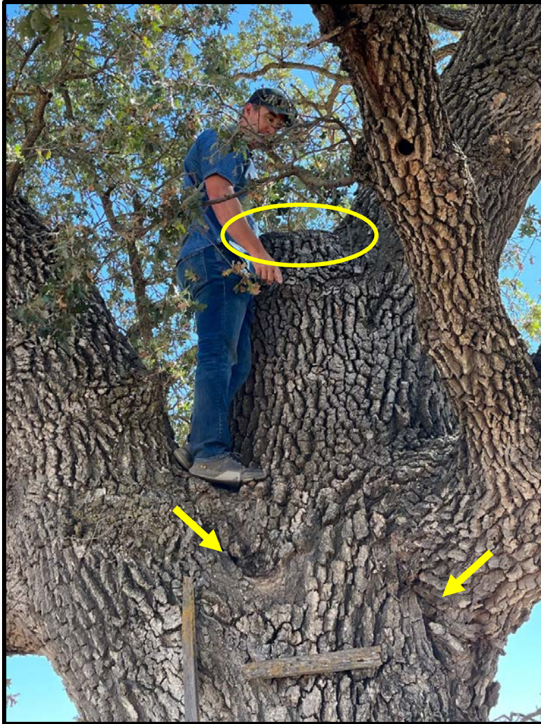
Photo 10 - Tree 2 perspective view of decay cavity formed by failed scaffold circled at center of tree. Cavity is circled. Other decay points below the open cavity are indicated by arrows.
