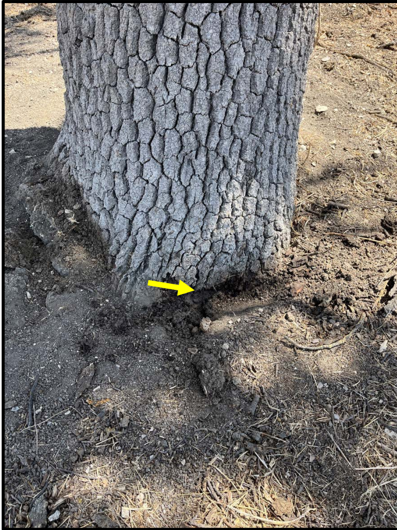
Photo 24 - Tree 11 close up of root crown decay at southwest side of tree indicated by yellow arrow. Ant nest discovered here which indicates dead and rotting wood.
