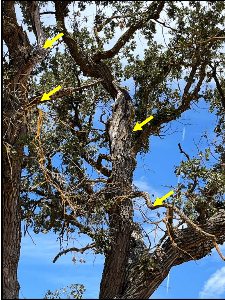
Photo 23 - Tree 11 close up of declining canopy, decayed branches, and dead wood indicated by arrows.
