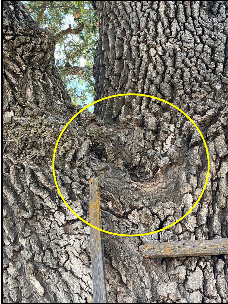
Photo 7 - Tree 2 with decay cavity at scaffold union approx. 8' above ground on southwest side of tree.
