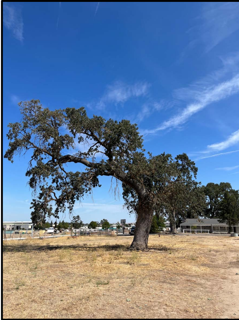
Photo 15 - View of Tree 3 to north. Overextended scaffold to west. Large decay cavity at connection to trunk.
