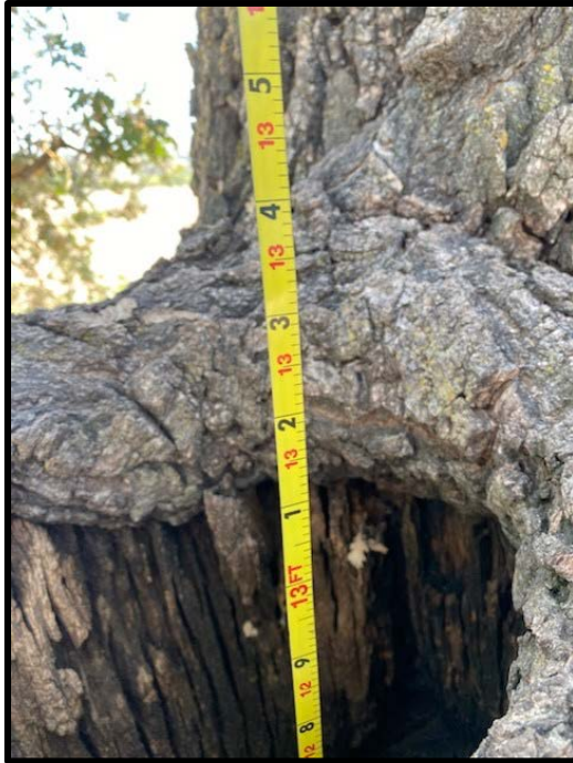
Photo 13 - Tree 2 measurement of interior depth of decay cavity formed by failed scaffold. 13' 2"
