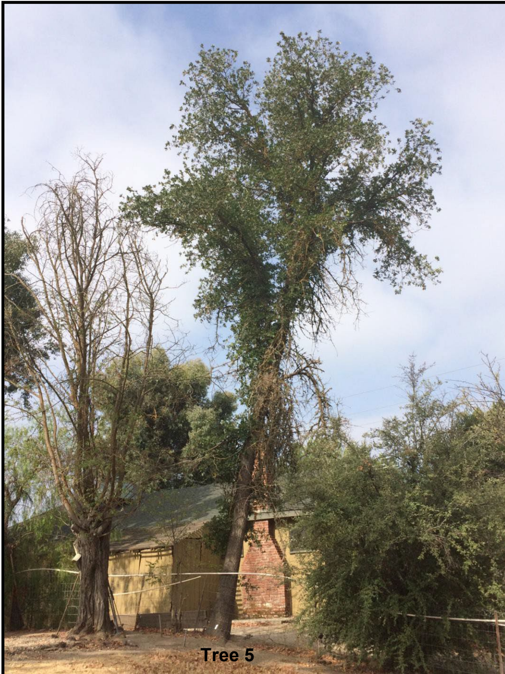
Photo 5 - View southwest of Tree 5 - Note drought stress indicated by dead branches and sparse canopy. Tree is outside property line.
