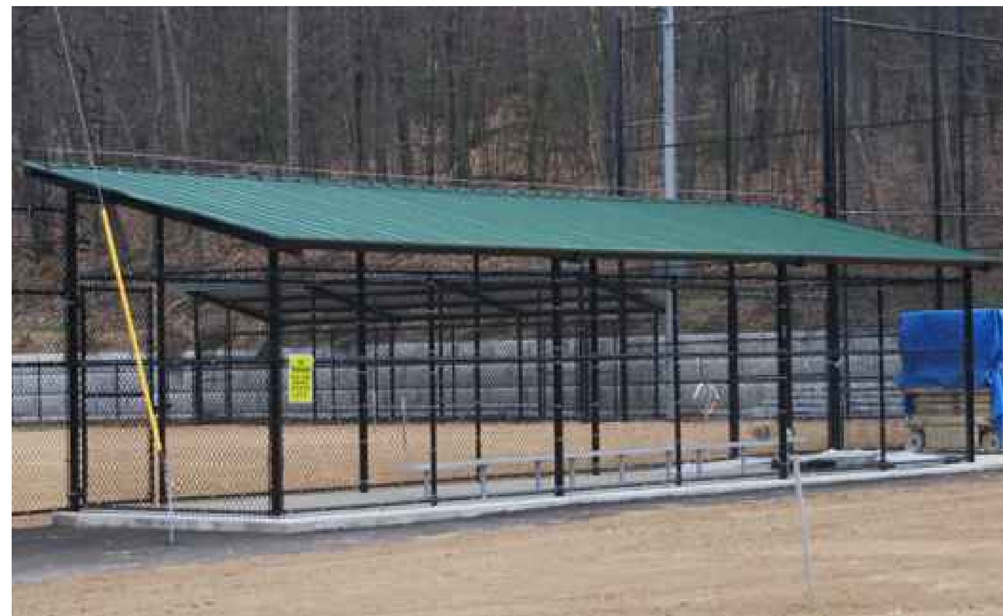
DUGOUT SHADE STRUCTURE
