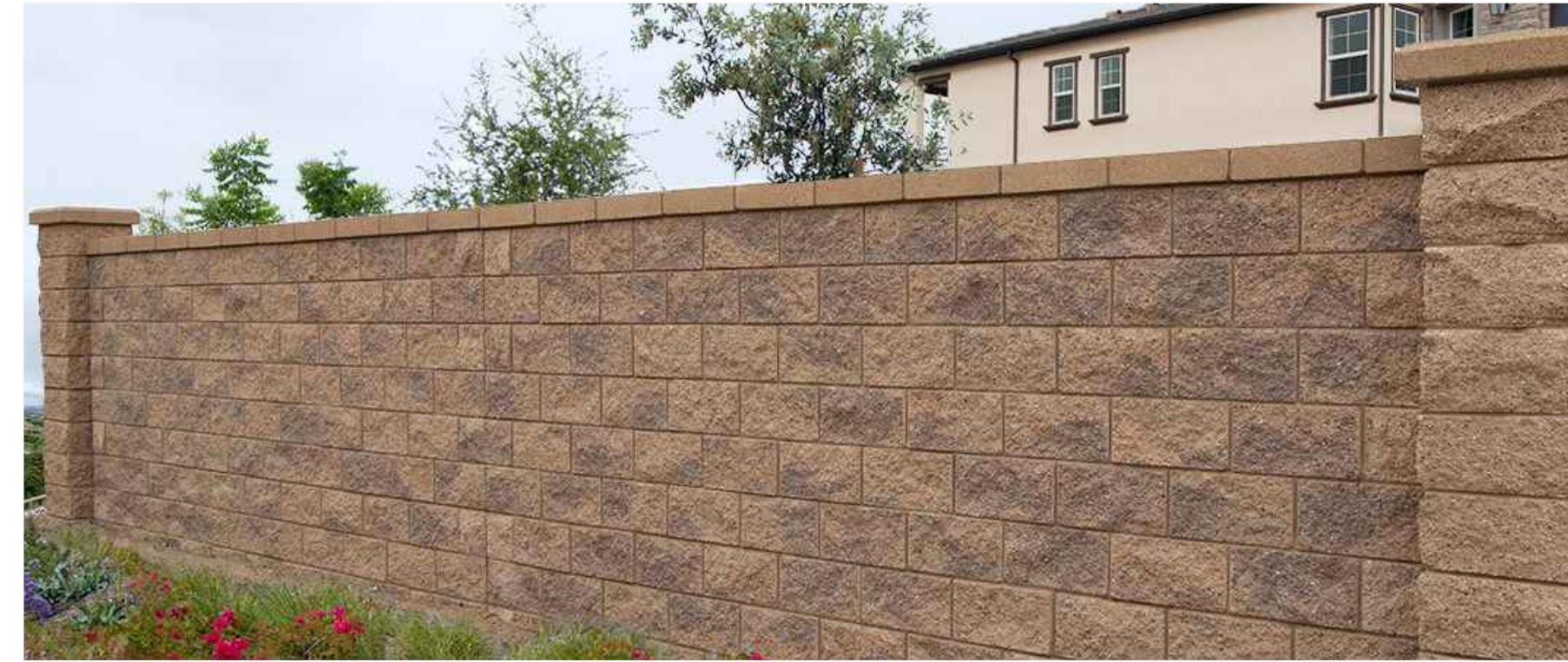
SPLIT FACE PERIMETER WALL
